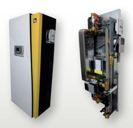
The **iDM fresh water station** can either be mounted **directly on the Hygienik or on the wall**.
