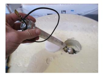
After the installation of the chain anode the drained water must be refilled. Before restarting the system, the buffer must be checked for leaks in the area of the protection anode.
