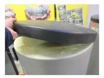
The foam, which serves as insulation in the area of the protective anode, must be removed.
