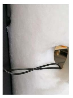
When the sensors are fixed, the insulation is closed again and the cover cap is attached. The cover also serves to provide a firmer hold of the sensor cables.
